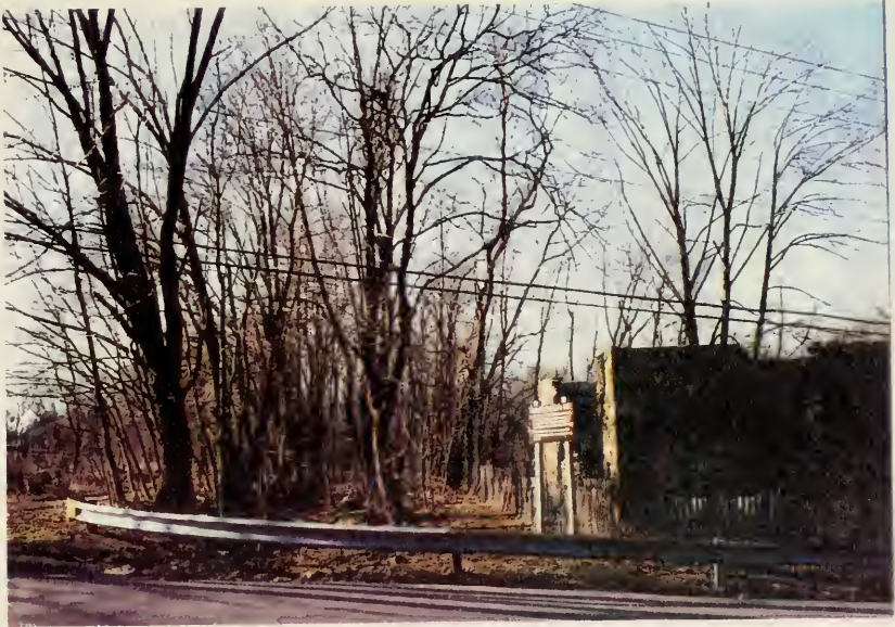
Fig. 14 Rapp's Dam mill race on the French Creek in East Pikeland Township, now abandoned. Photograph by the author, 1994.
